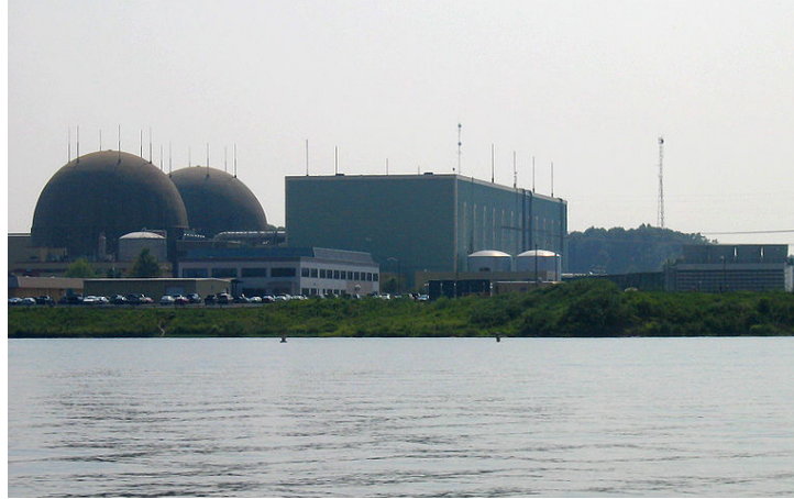
North Anna Nuclear Power Station / Photo: Dominion Power
